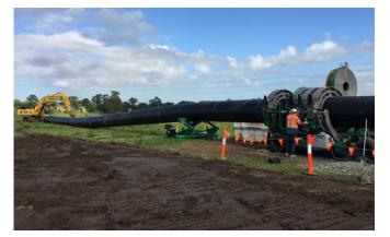
Onsite installation of the dual 1200mm PN16 polyethylene pipeline.
